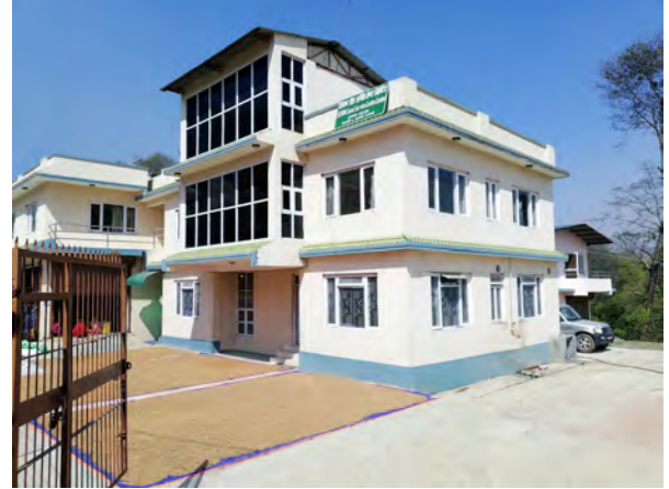
Office building at Thankot, Kathmandu
